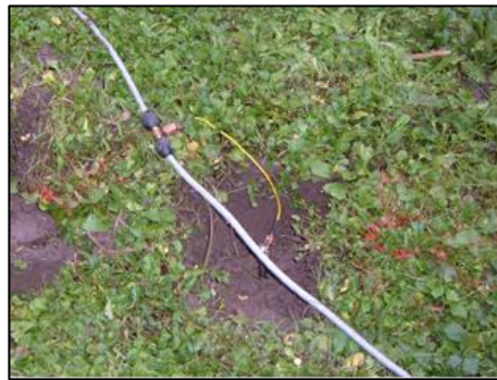
Figure 3. Connection of electrodes with equipment by cable
